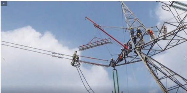
Hot line maintenance activities in EHV electrical sub-station and transmission line
