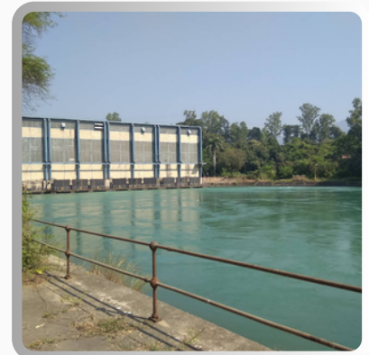
GANGUAL CANAL POWER HOUSE
